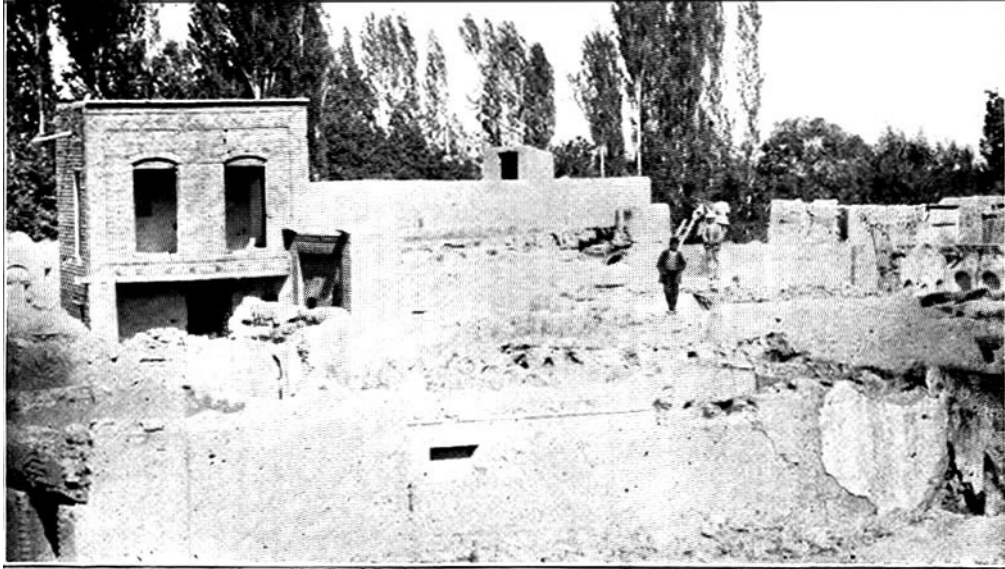
THE ONLY HOUSE REMAINING IN WAZERABAD
